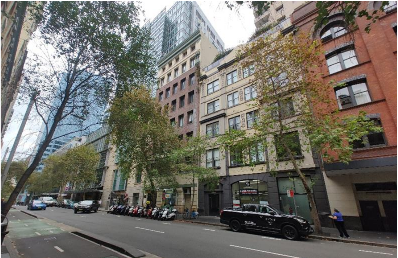
Figure 9 – Kent Street, general view facing south-east Source: Urbis, March 2023
