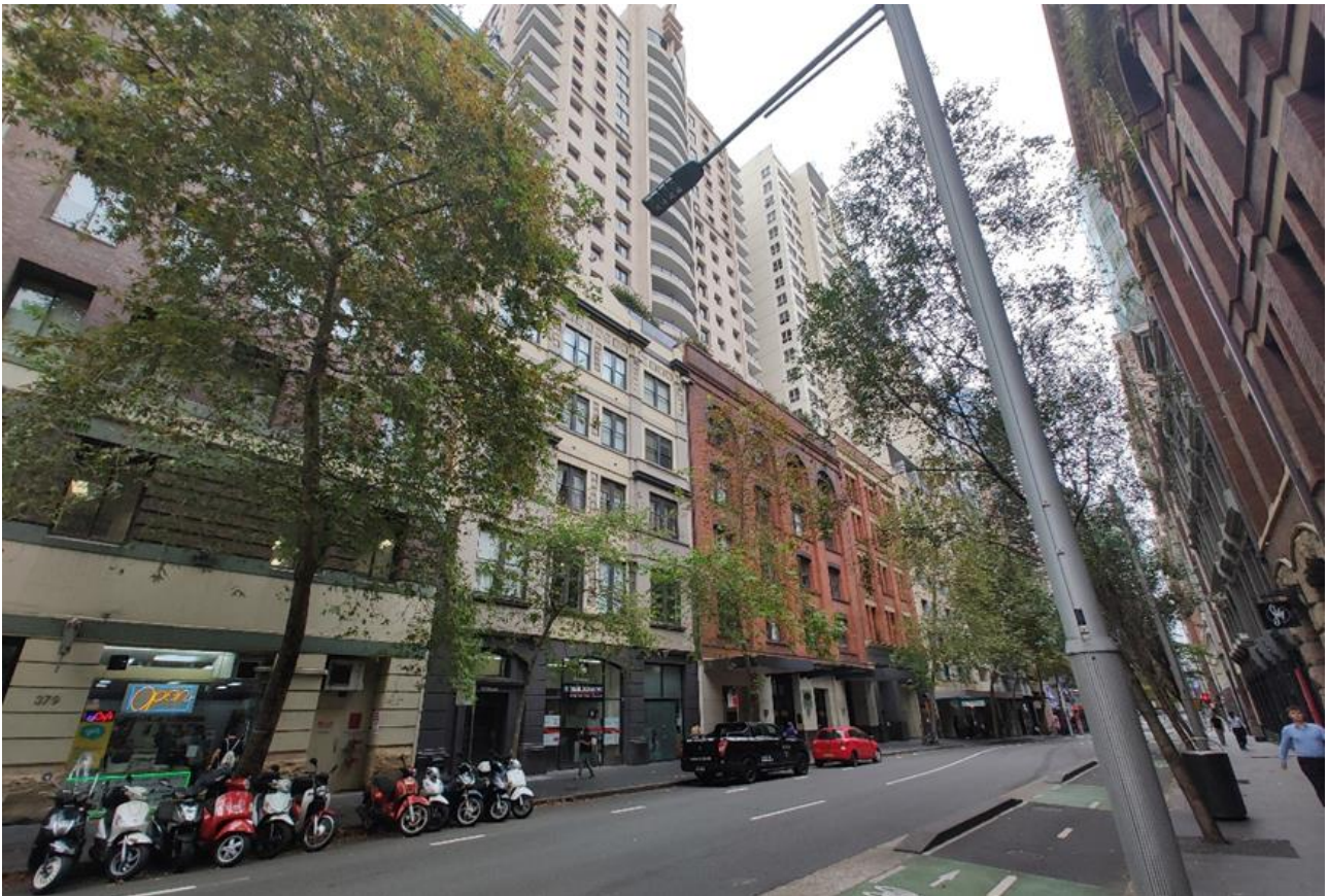
Figure 8 – Kent Street, general view facing north-west Source: Urbis, March 2023
