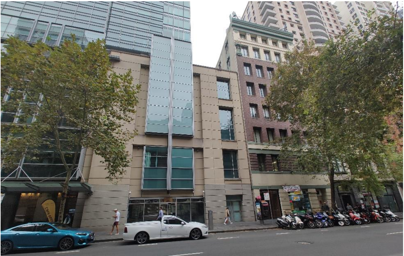
Figure 7 – The boundary between the subject site and neighbouring building on the north side Source: Urbis, March 2023
